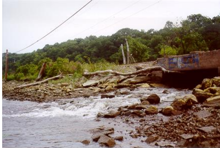
FIGURE 5. Looking into Suckley Cove culvert at low tide; the invert is above the river water level.
